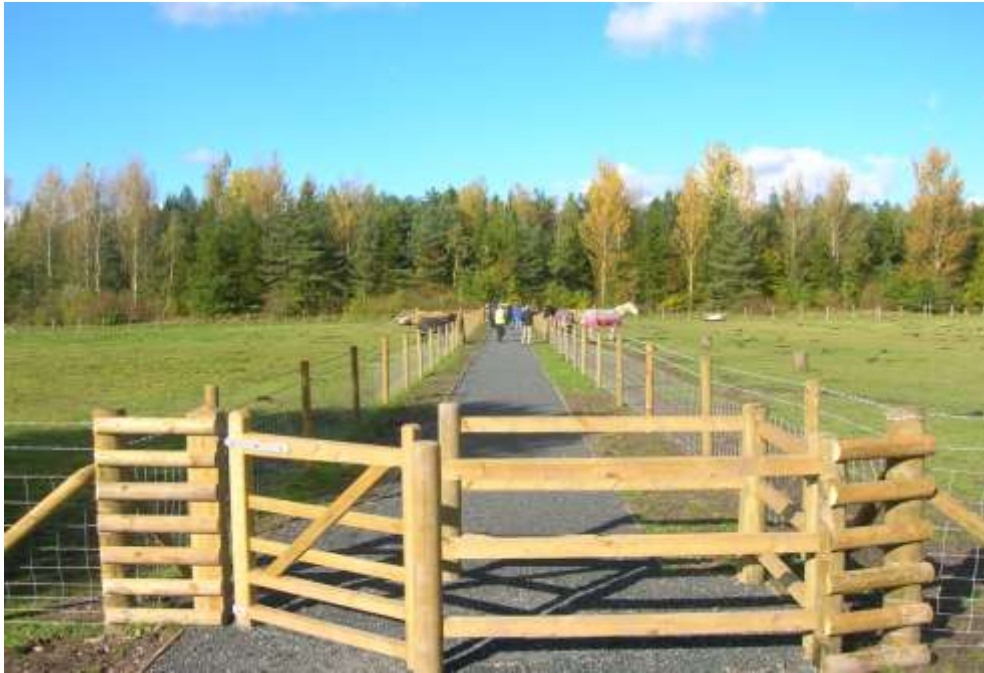
Rough Park, Woodside, Telford: TATN funded 100m accessible path
