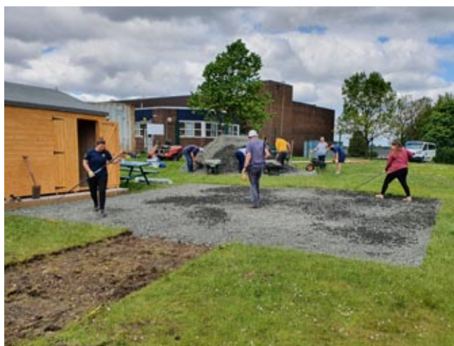
Laying down Type 1 hardcore as the base for raised beds. DAVID MACDONALD
