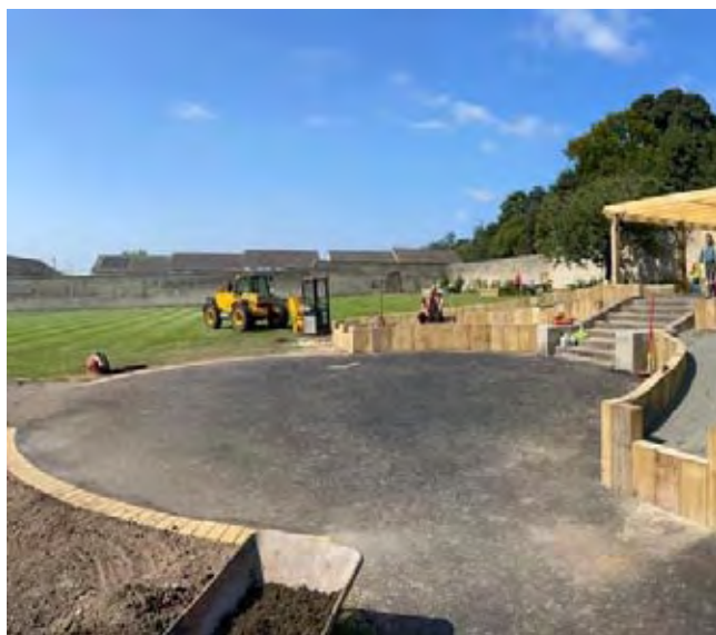
The amphitheatre under construction. DONNA MCLEAN
