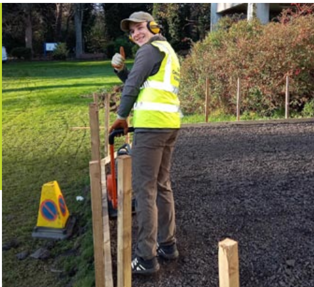
VO Joe Churchill using a wacker plate.
