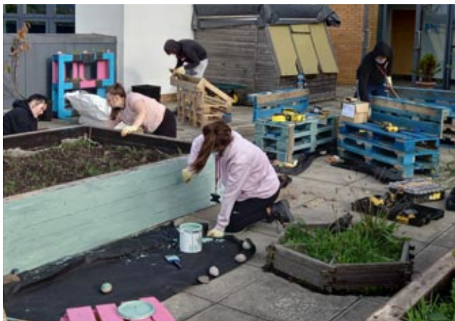
Painting a planter On the Roof.
