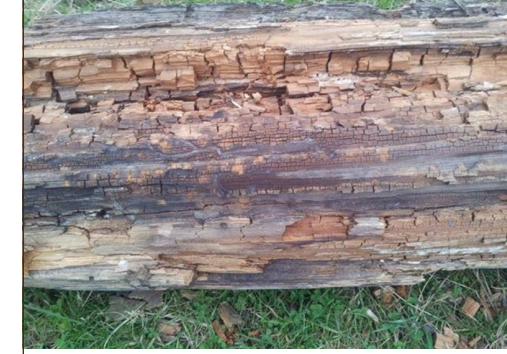
DECAY STAGE 2: Predators arrive
